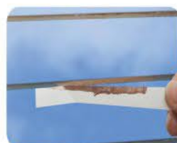
REMOVE THE MASKING TAPE IMMEDIATELY
