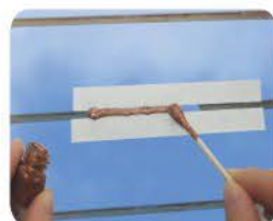
APPLY THE SILVER REPAIR COMPOUND IN BETWEEN THE TAPE
